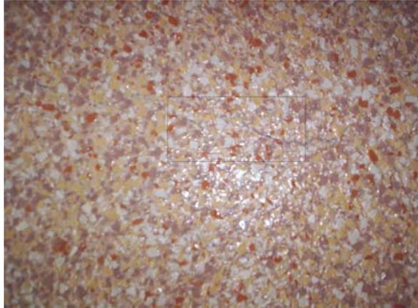
Deep cracks that are not filled before application may appear through the flake system. These areas may be patched over to hide the distinctive black line.
